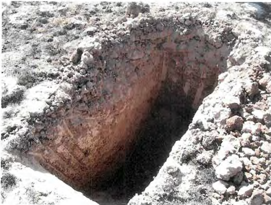
Figure 6. View of 6-foot excavation pit dug in Northwest Area by 253 rd Engineer Detachment.
